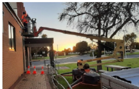
Above: Gutter cleaning and tree trimming completed at the Taillem Bend Town Hall.
