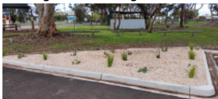
Above: New plants and gravel installed, Coonalpyn swimming pool car park area.
