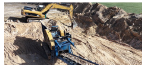
Above: Crushing at rubble pit on Taunta Hut Road.
