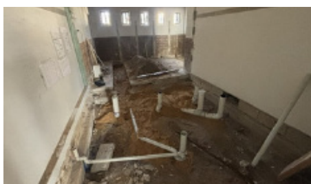
Above: Demolition works completed & plumbing trenching commenced at Tintinara War Memorial Hall
