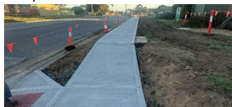
Above: First completed portion of the concrete footpath works, Meningie.
