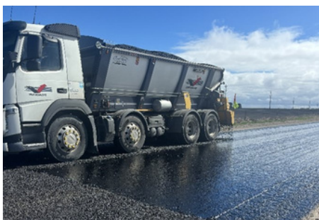
Above: Spray seal works, Narrung Road.
