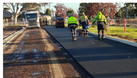
Above: Hotmix asphalt works at Railway Terrace Carpark, Taillem Bend
