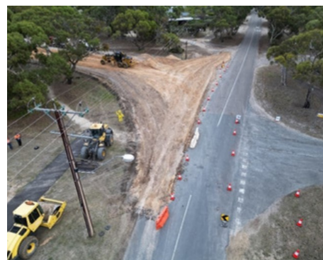
Above: Progress photos of the Northcott Avenue works underway.
