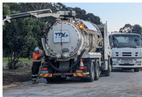
Above: SA Water connecting to existing Council infrastructure at Wellington East.
