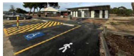
Above: Carpark and footpath works completed at Coonalpyn.
