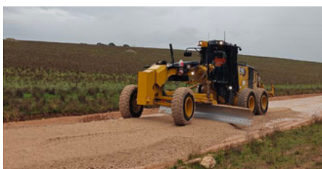
Above: Final trimming works occurring at Buccleuch North Road, Peake
