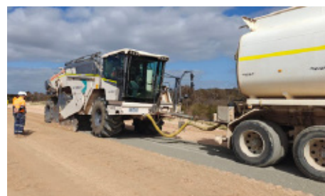
Above: Cement stabilisation works underway for Carcuma Road upgrade.
