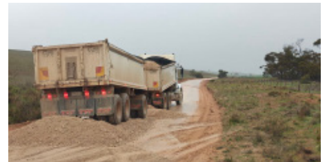
Above: works underway on Buccleuch North Road at Peake.
