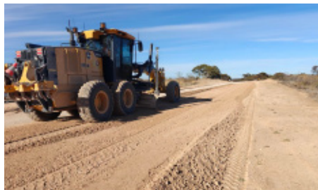
Above: Final trimming works of base course layer for Carcuma Road Stage 2B.
