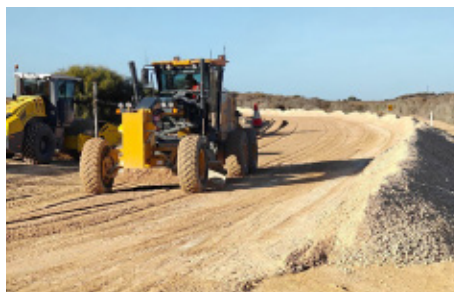
Above: Subbase layer construction underway at Carcuma Road, Tintinara.
