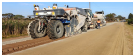
Above: Cement stabilisation on Alexandrina Drive, Narrung.
