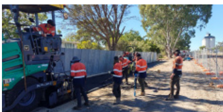
Above: Laying asphalt footpath, Fulwood Avenue to the Tintinara Apex Park
