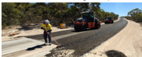
Above: Spray Seal works on Carcuma Road, Tintinara.
