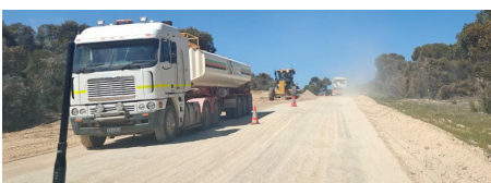
Above: Subbase being shaped and moisture conditioned at Carcuma Road, Tintinara
