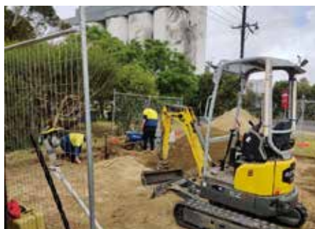
Pictured above: Civil works being carried out to set up an EV charging station at Coonalpyn
