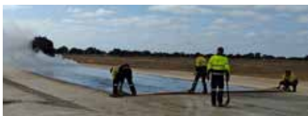
Pictured above: Spray-seal works for primary runway at Tintinara Airport
