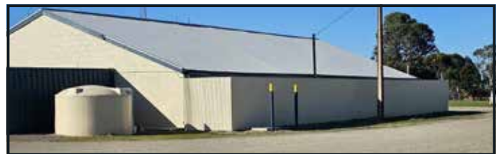
ABOVE: Western side after renovation.
