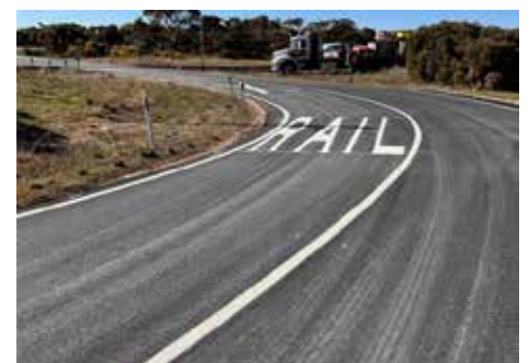
Above: Line-marking & pavement message completed on Frost Road railway crossing.
