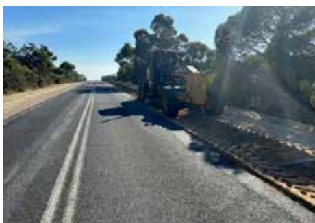
Above: Carcuma Road shoulder compaction prior to sealing.
