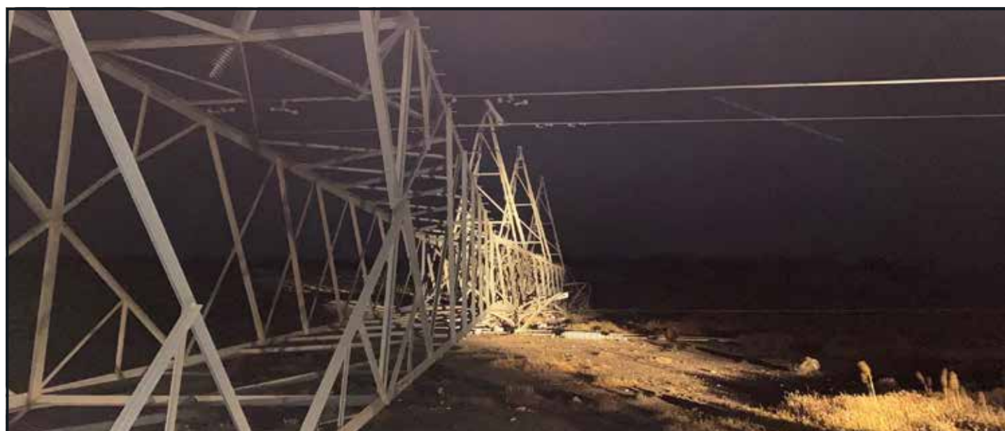
ABOVE: ElectraNet, image from Facebook. On November 12th a significant weather event damaged a transmission tower just outside Tailem Bend. Customer supply has not been impacted.
